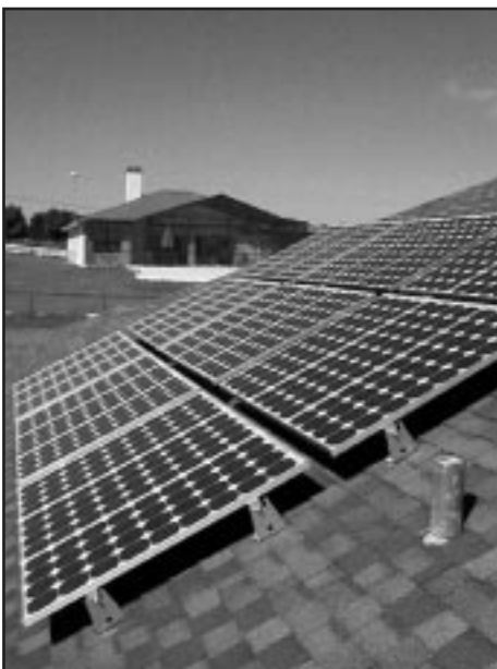
A super energy-efficient PV home in Lakeland, Florida. On the bar graph, the control home represents a typical Florida home, and used 37.5 kWh on a sunny day in May. On the same day, the energy-efficient PV home used only 5.8 kWh (84% less than the control) and sent net power back to the utility. The solar array produced 17.9 kWh, almost three times what was used.
