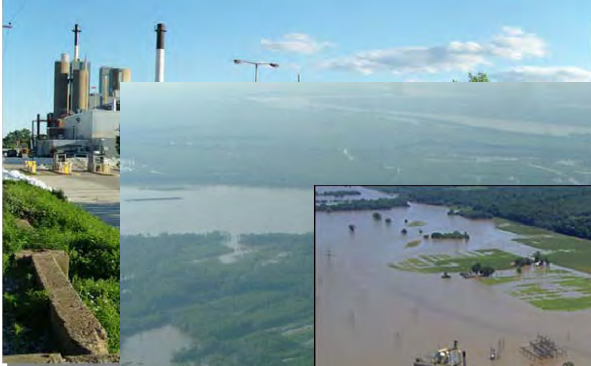
U. Iowa Plant 2008 Flood. Source: Flickr
