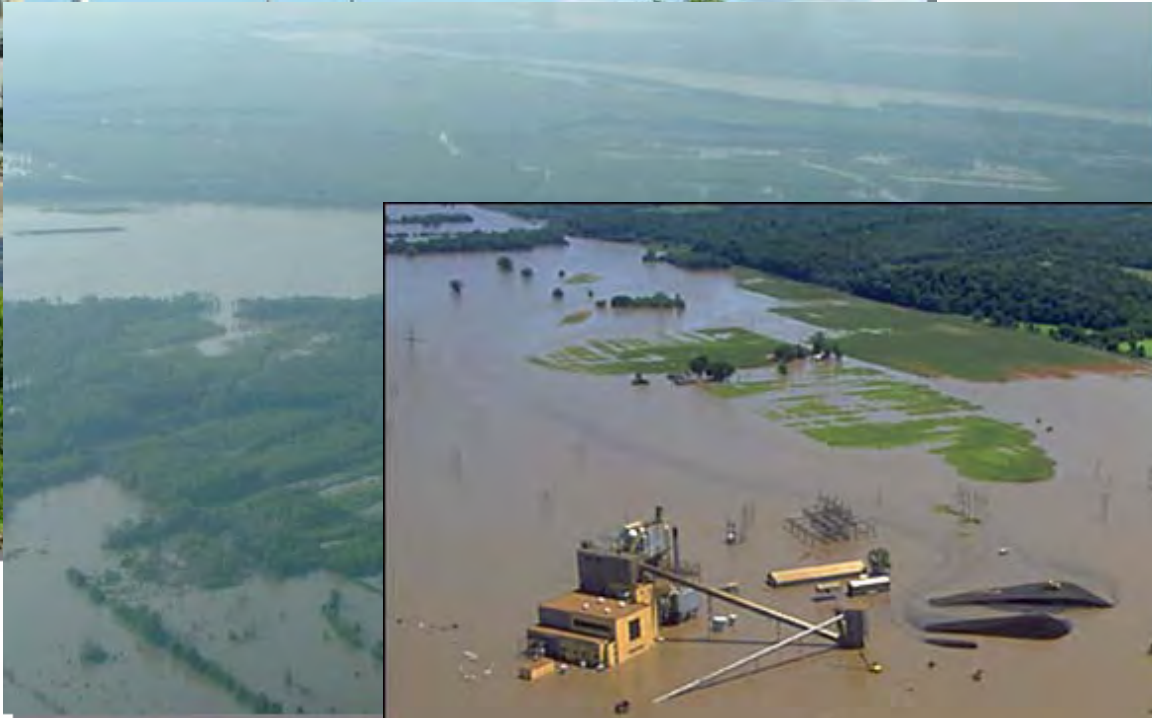
Baxter Wilson Power Plant, April 2008. Source: Flickr
