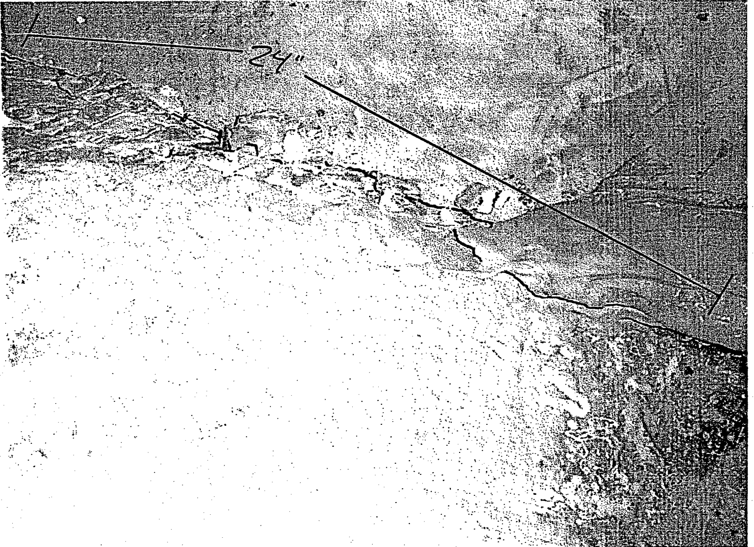
24" Floor Cracking to the left of the manway.
